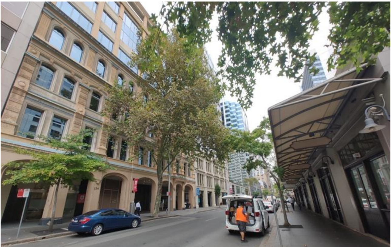
Figure 14 – Sussex Street, general view facing south-east, showing façade of listed warehouse building at left of frame Source: Urbis, March 2023
