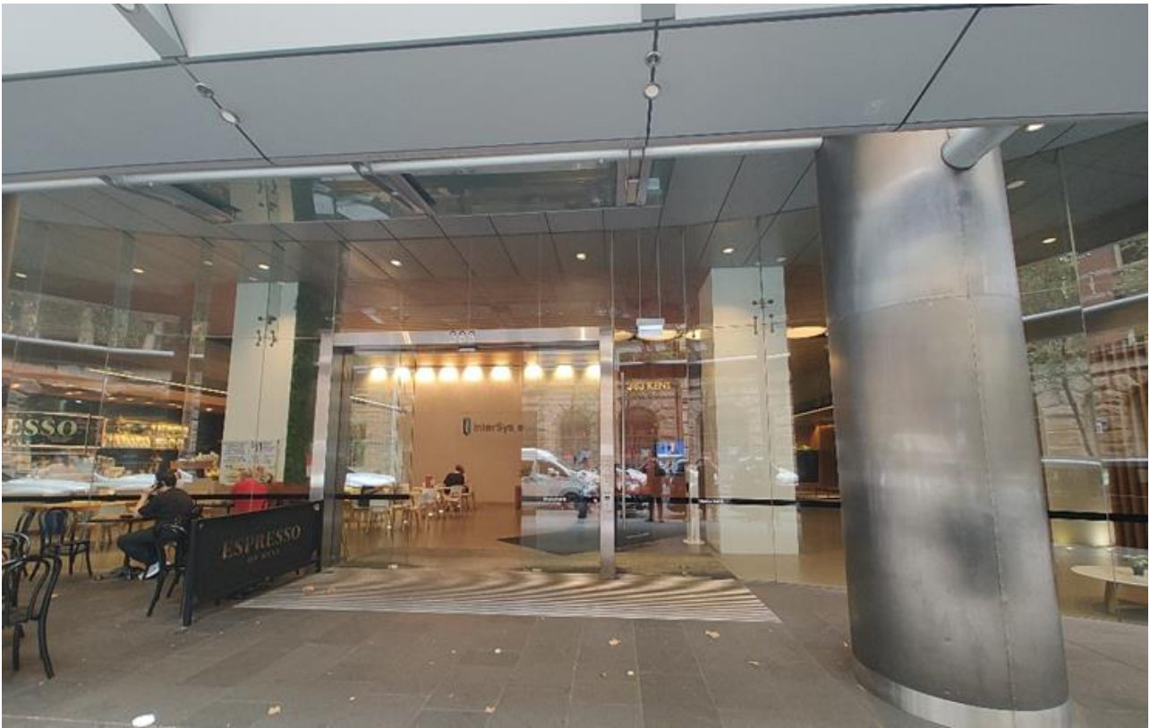
Figure 18 – Front lobby and small retail tenancy at ground-floor level of subject building, at Kent Street Source: Urbis, March 2023
